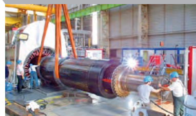
Site service - generator disassembly
