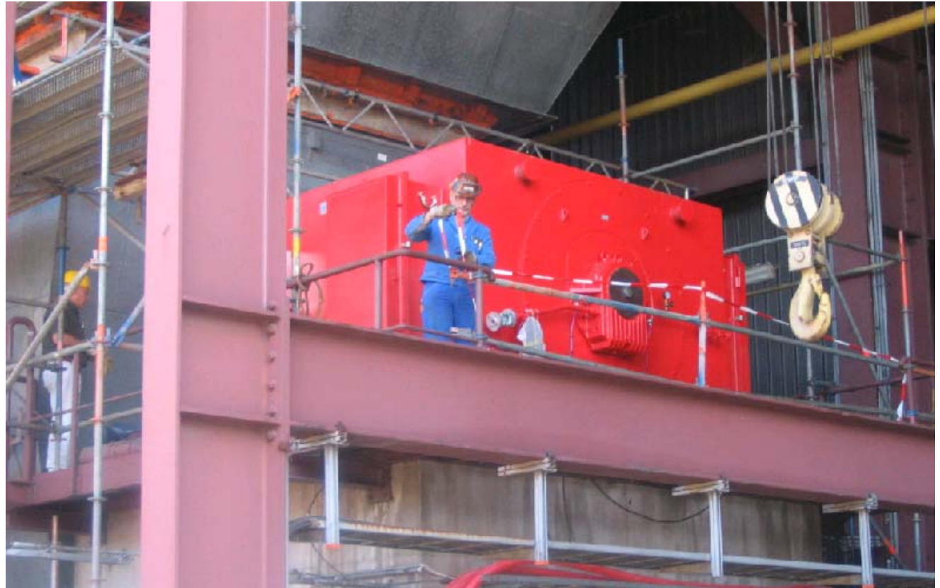
Coal fired power plant
