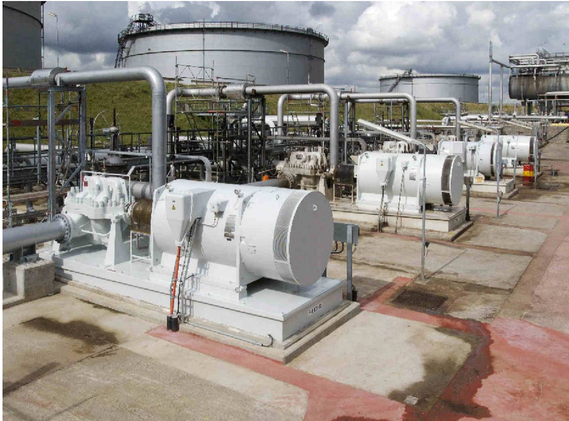
Drive for crude oil pumps, EExd(e) IIB T4, 1,500 kW, 10 kV, 1,490 rpm
